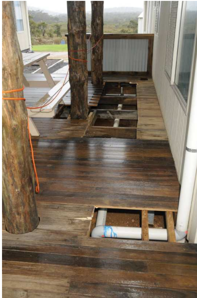
Photograph 1 - The deceased was working on the drainpipe depicted in the foreground
