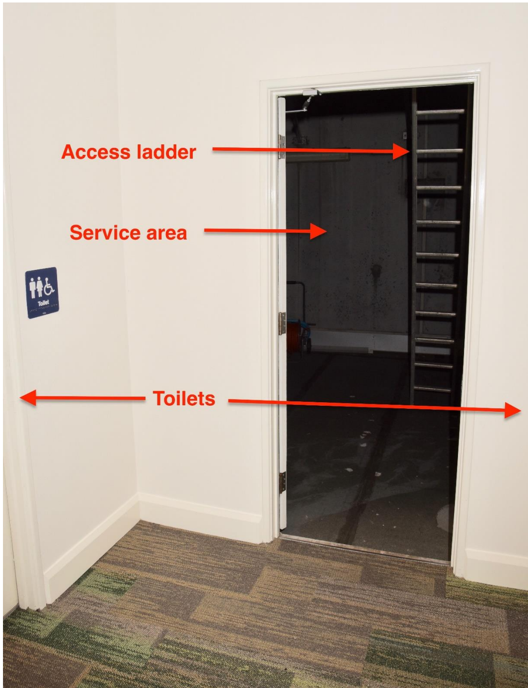
Photo 2: Shows the service area and the right-hand toilet door. 33
