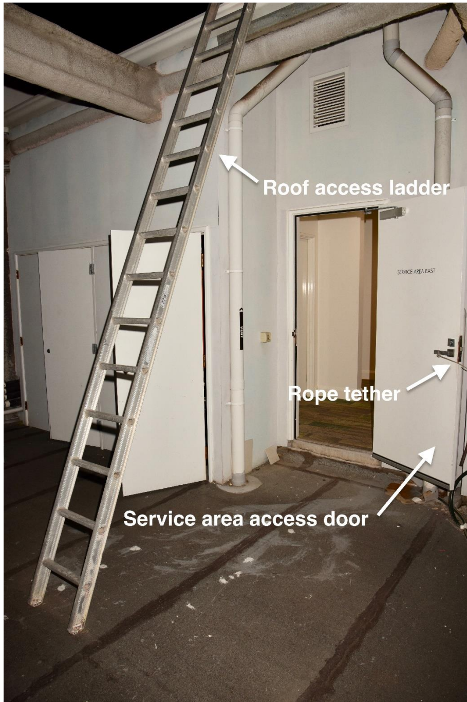
Photo 3: Access door to service area and roof access ladder 34
